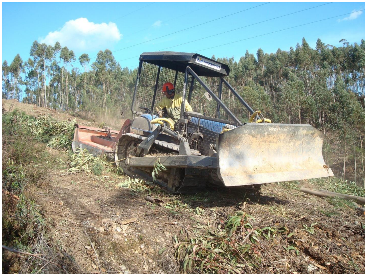
Bulldozer clearing a fuel break in a eucalyptus forest. Photo Credit: Vasco Campos
