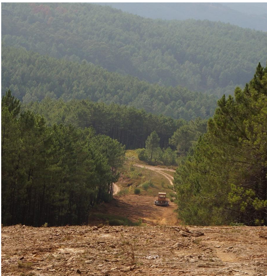
Photo 4: Bulldozer break being cleared – up and down the slope!! This is really not environmentally sound as it will cause erosion.
